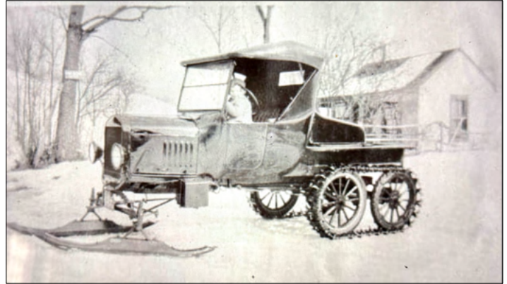
Jim Benzie modified his 1915 Model T Ford to carry the mail and equipped it with Page chains for both winter and mud season use. He also purchased a Snow Flyer Conversion Kit so he no longer had to use the horse and sleigh in the winter and could rely just on the Model T.
