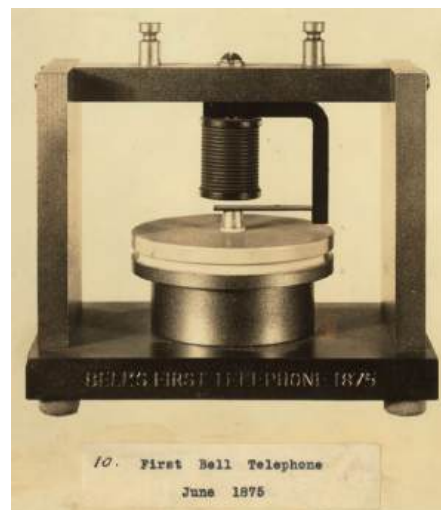
The first telephone, made by Alexander Graham Bell in 1875. The telephone, i regarded as an amusement, initially struggled to compete against the telegraph. Photograph from the Library of Congress.
